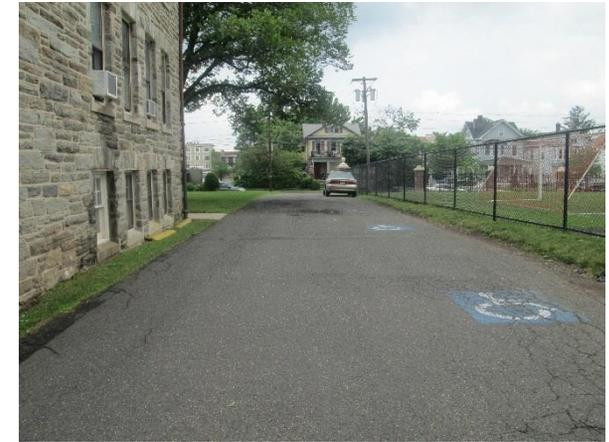
Parking spaces adjacent to the rear of the church can be replaced with pervious pavement to infiltrate stormwater. Bioretention systems can be installed to capture roof runoff by disconnecting and redirecting two nearby downspouts. A preliminary soil assessment suggests that the soils have suitable drainage characteristics for green infrastructure.
